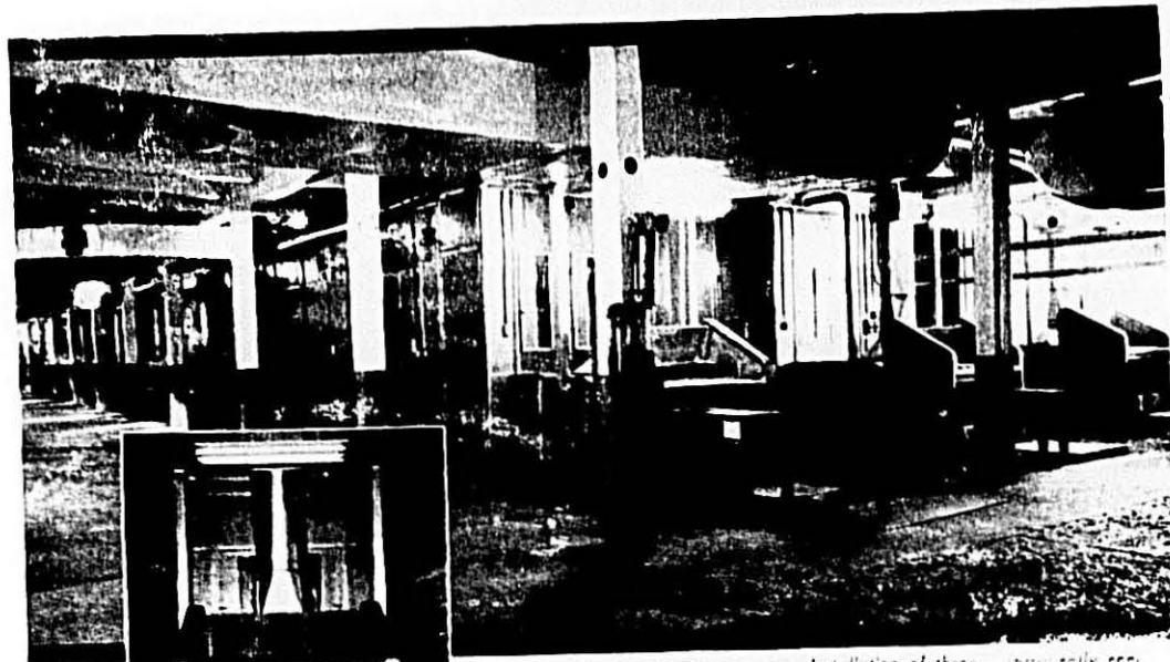
Installation of three automatically controlled Long Goods Dryer Units at Cattelli.
